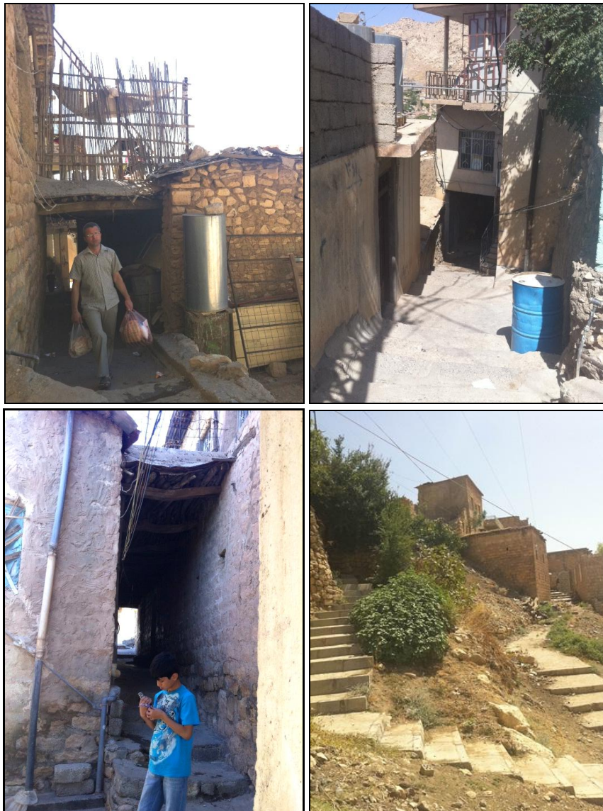
Figure 8-21: Different mode of historic houses connection and space sharing in Akre City
