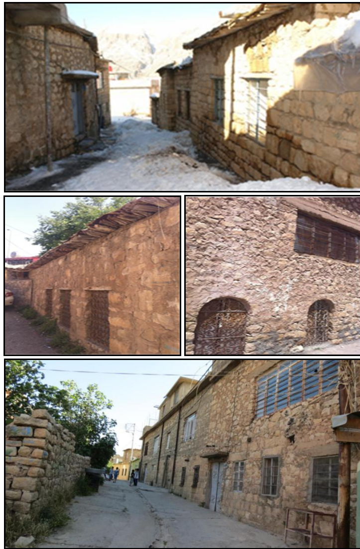
Figure 9-26: Examples of building style in Amedy city Source: Own Photos, 2011
