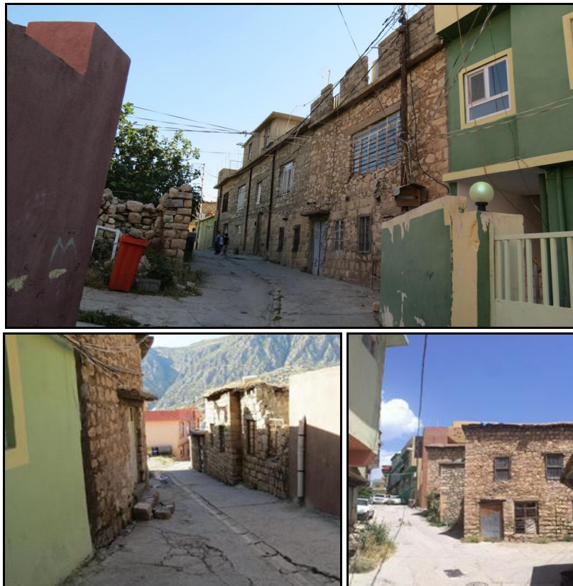
Figure 9-29: Poor physical condition of traditional buildings in Amedy city, some are replaced by new buildings
