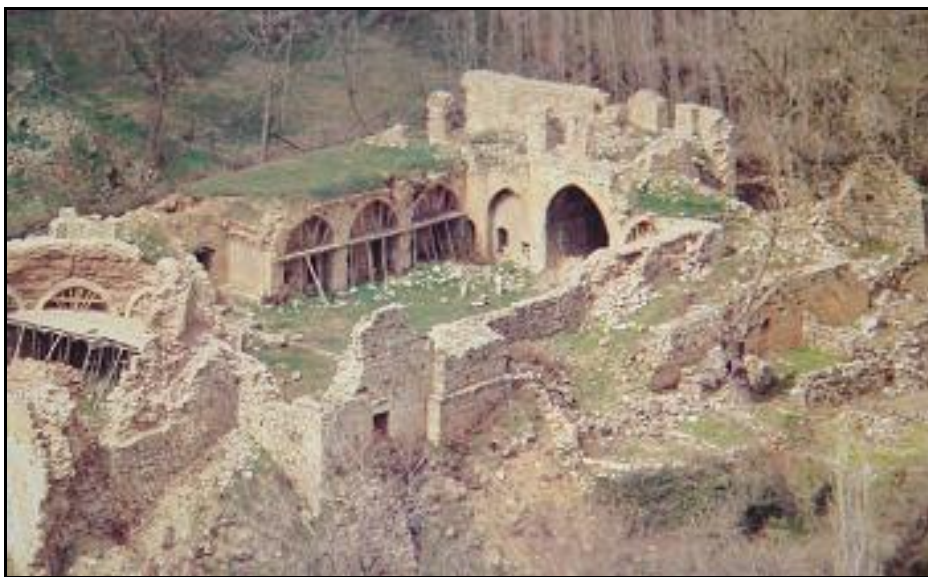
Figure 9-37: Poor conditions of Qubahan School in Amedy city Source: Own Photo, 2012
