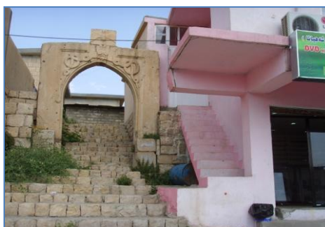
Figure 9-34: Uncontrolled changes affecting Bahdinan Emirate Symbol Source: Own Photos, 2012
