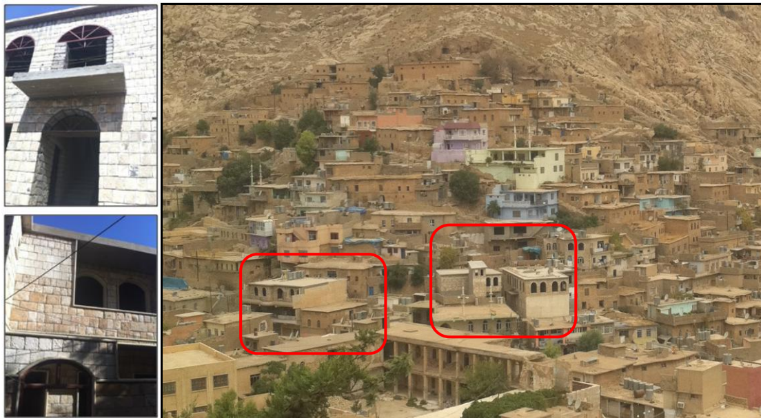
Figure 8-33: Houses reconstructed by Akre Municipality
