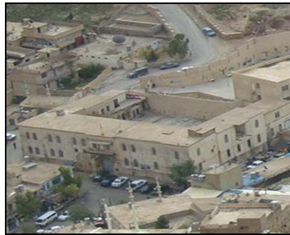
B. Northern side of Qishla building
