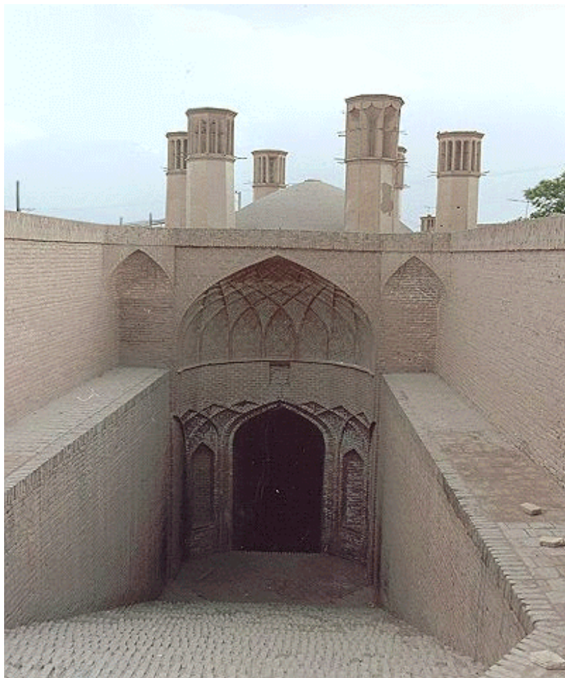
Figure 49: Stairway and windcatchers of an Ab-anbar in Yazd (Source: (Alfaee 2009))
