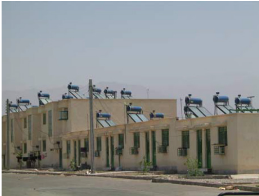
Figure 103: Solar Water Heaters in Jiroft (Source: mehr-abad.ir)
